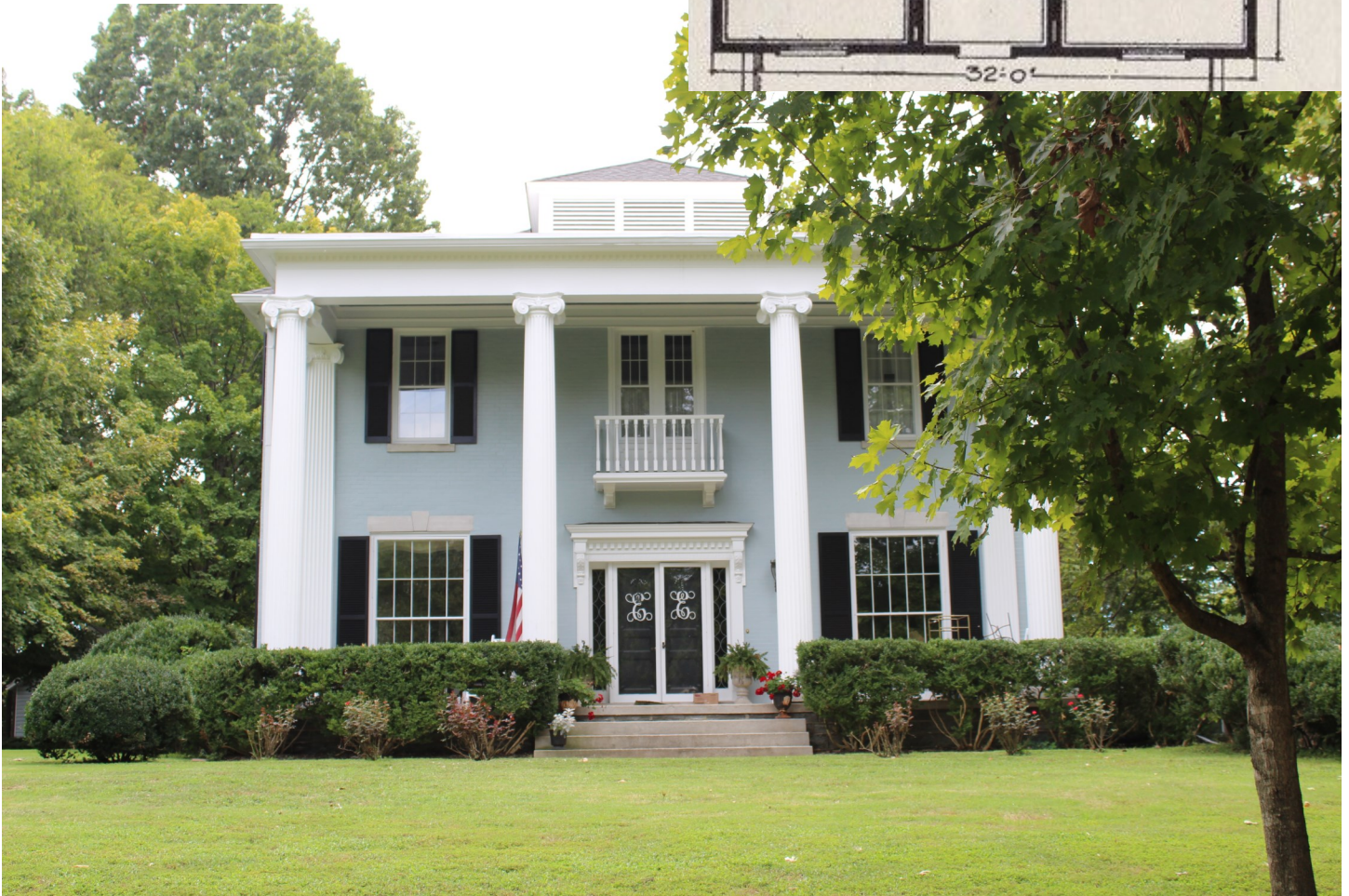
The Davis-Esslinger Home on West Seventh Street. Above that is a floor plan for foursquare Model No. 264B102.
